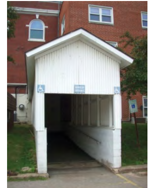
Covered rear entrance ramp
