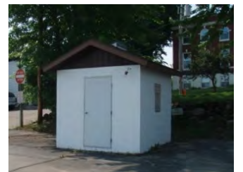
Onsite well/well building
