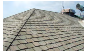
Roof in good condition
